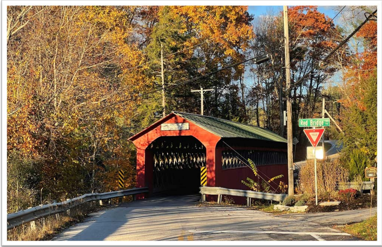
The historic Chiselville Covered Bridge
