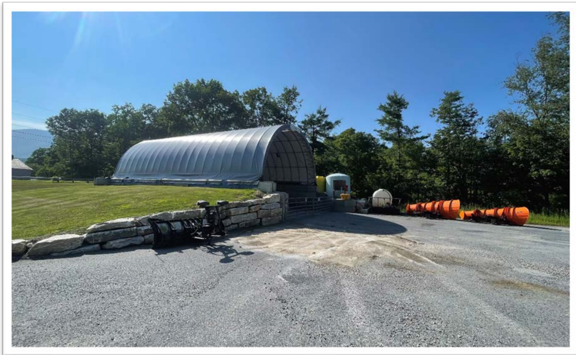
Salt shed at Town Garage
