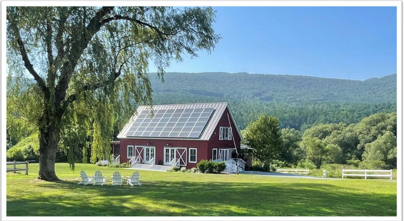
Solar power generation at Hill Farm
